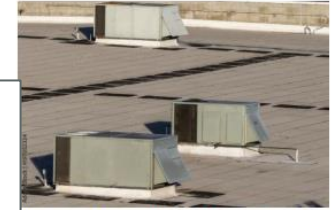
Packaged rooftop units (RTUs) on commercial building roof. Source: Adobe Stock Images
